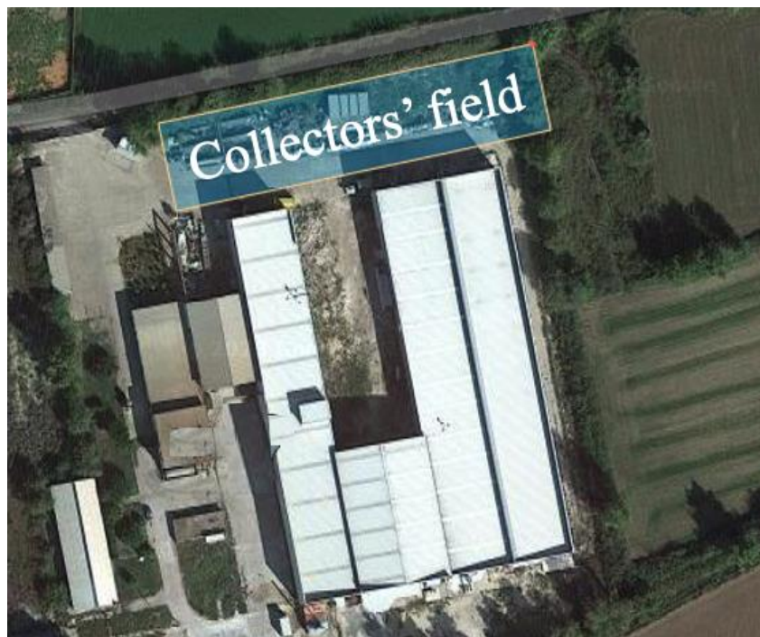
Figure 35: Solar field size in the installation
