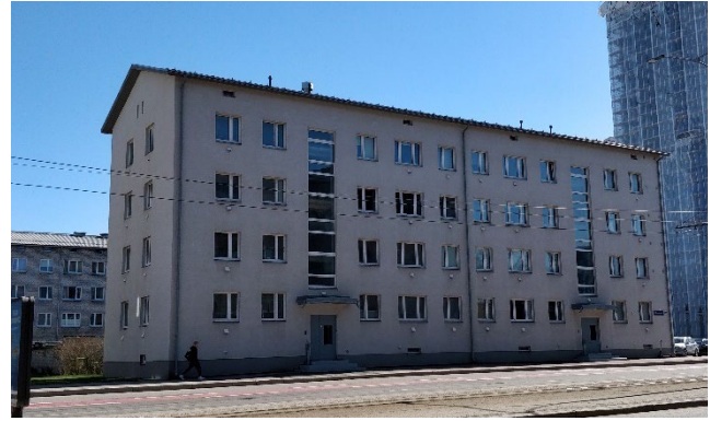
Figure 20: The renovated building, type 1-317
