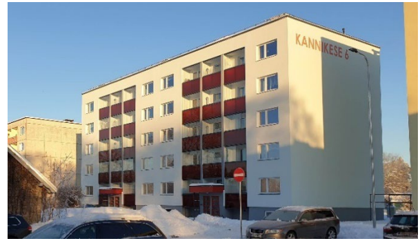
Figure 6: The renovated building, type 111-121
