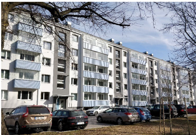
Figure 17: The renovated building, type 1-464
