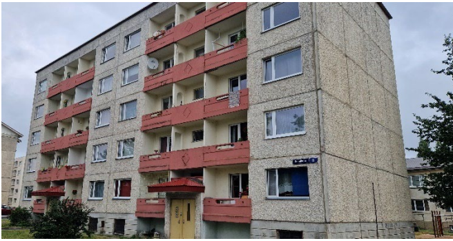
Figure 5: The original building, type 111-121
