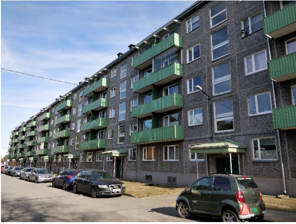
Figure 11: The original building A, type 1-464
