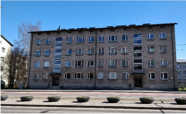
Figure 19: The original building, type 1-317
