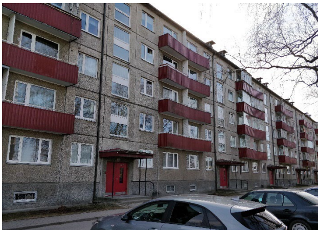
Figure 16: The original building, type 1-464
