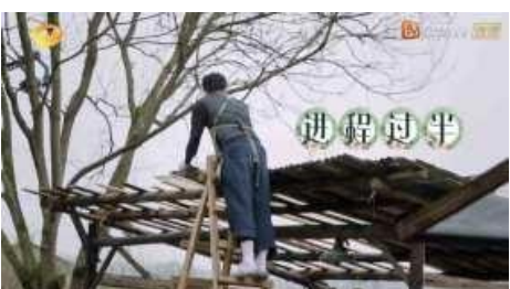
Building the Greenhouse (E3)
