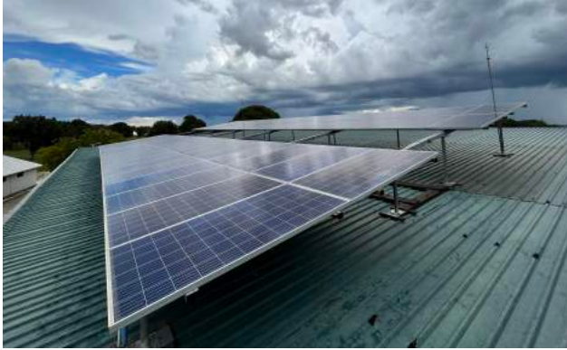
(a) Solar panel installation at St. Ann Catholic Mission Hospital.
