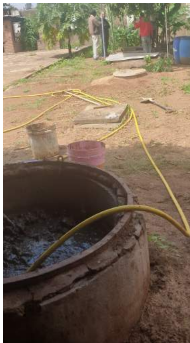
Figure 14: Biogas plant system at Site 1 (Lovisa Magnusson Ericsson, 2023).
