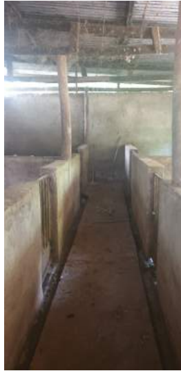
(a) Concrete stables for the pigs with a sloping floor toward the channels in the middle corridor. (b) Personnel sweeping the floor in the pig stables to manually collect the manure to use as substrate in the digester.
