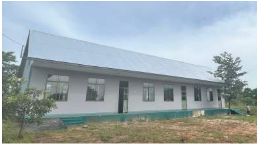
(a) Existing classroom building.
