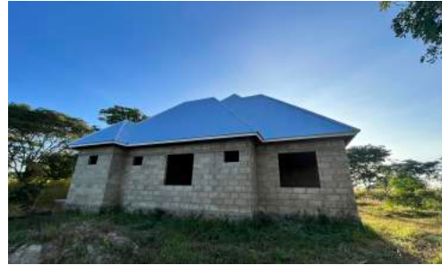
(b) Accommodation house (in progress).
