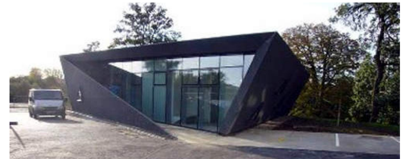
Maggie's center in Fife-Scotland by Zaha Hadid, finished 2006 Foto 11: / www.worldconstructionnetwork.com downloaded 2023
