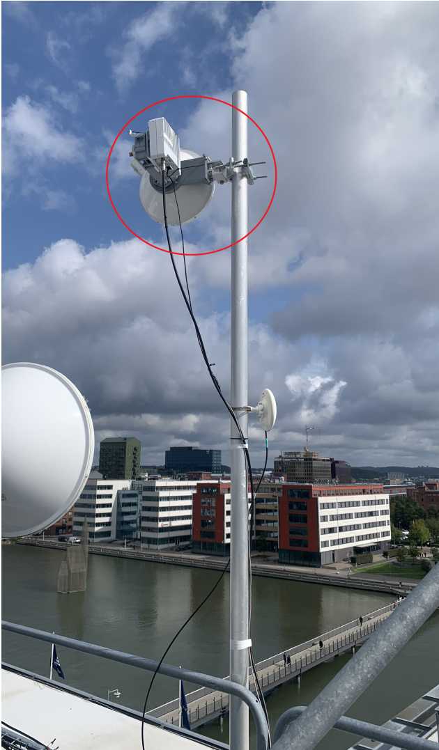
Figure 90: Mounting antenna-radio system on a pole
