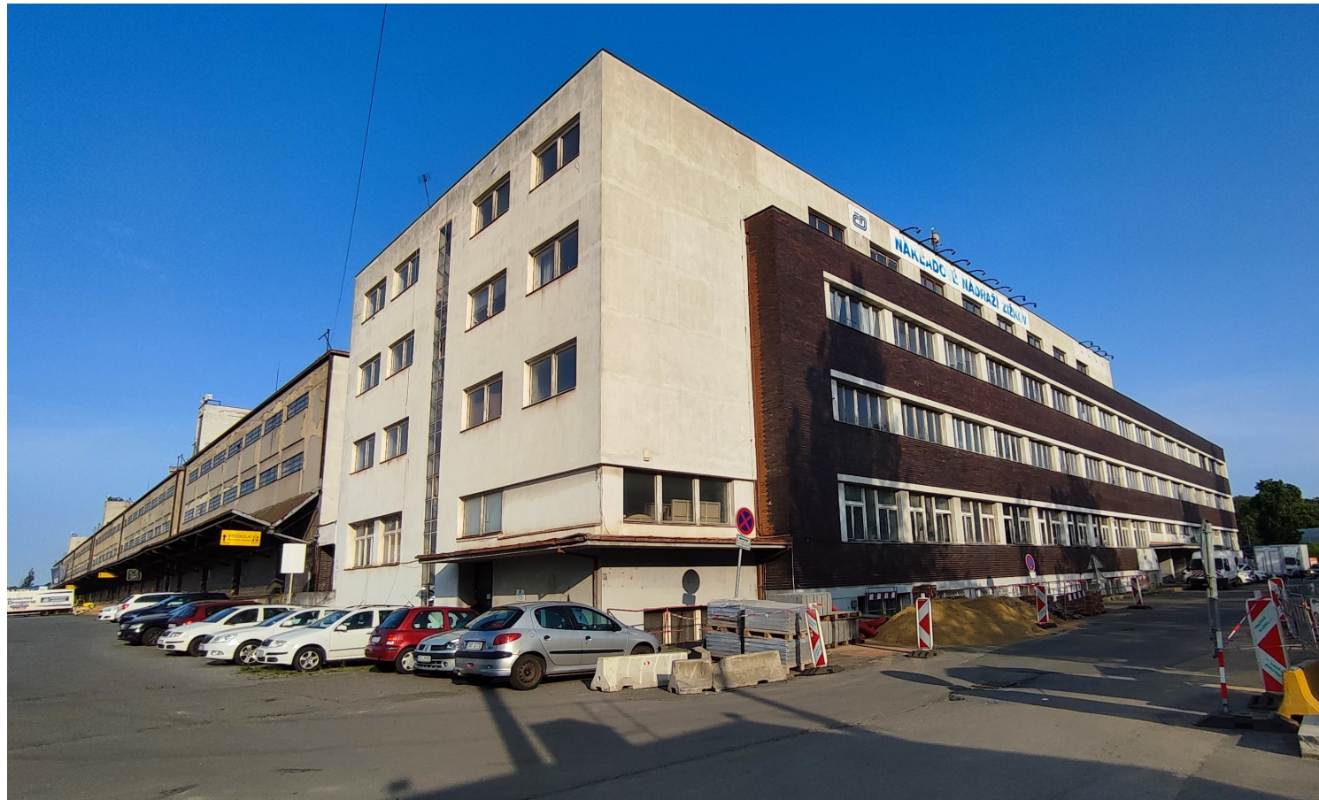
Image 22: Site view, administrative building in the center
