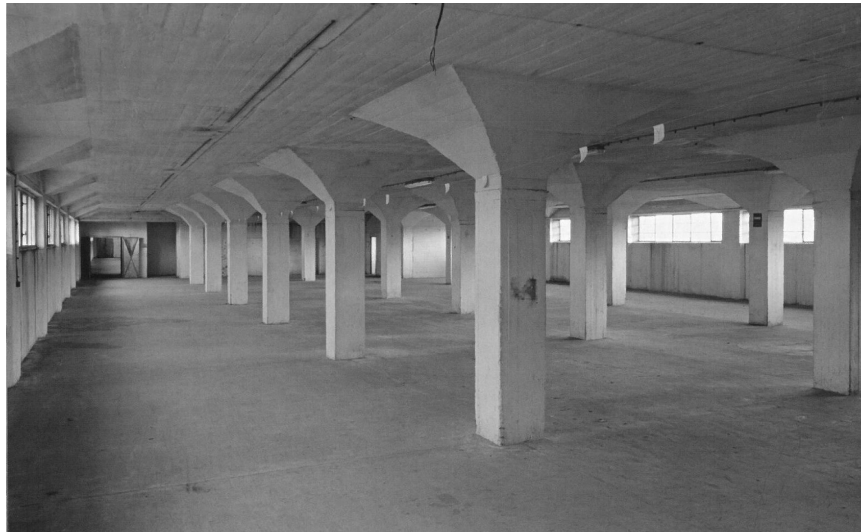
Image 31: Inside the Northern warehouse, second floor.
