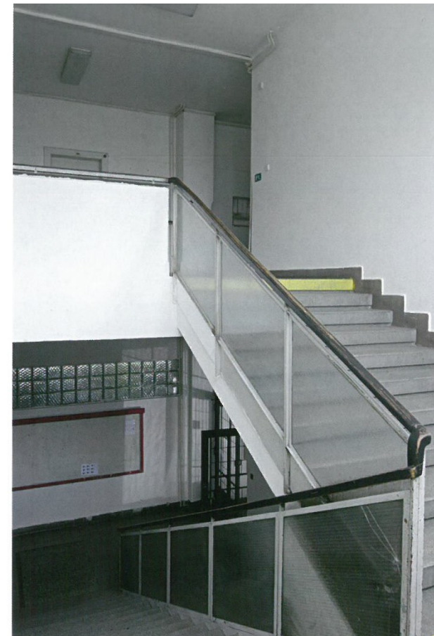
Image 23: Staircases inside the administrative building
