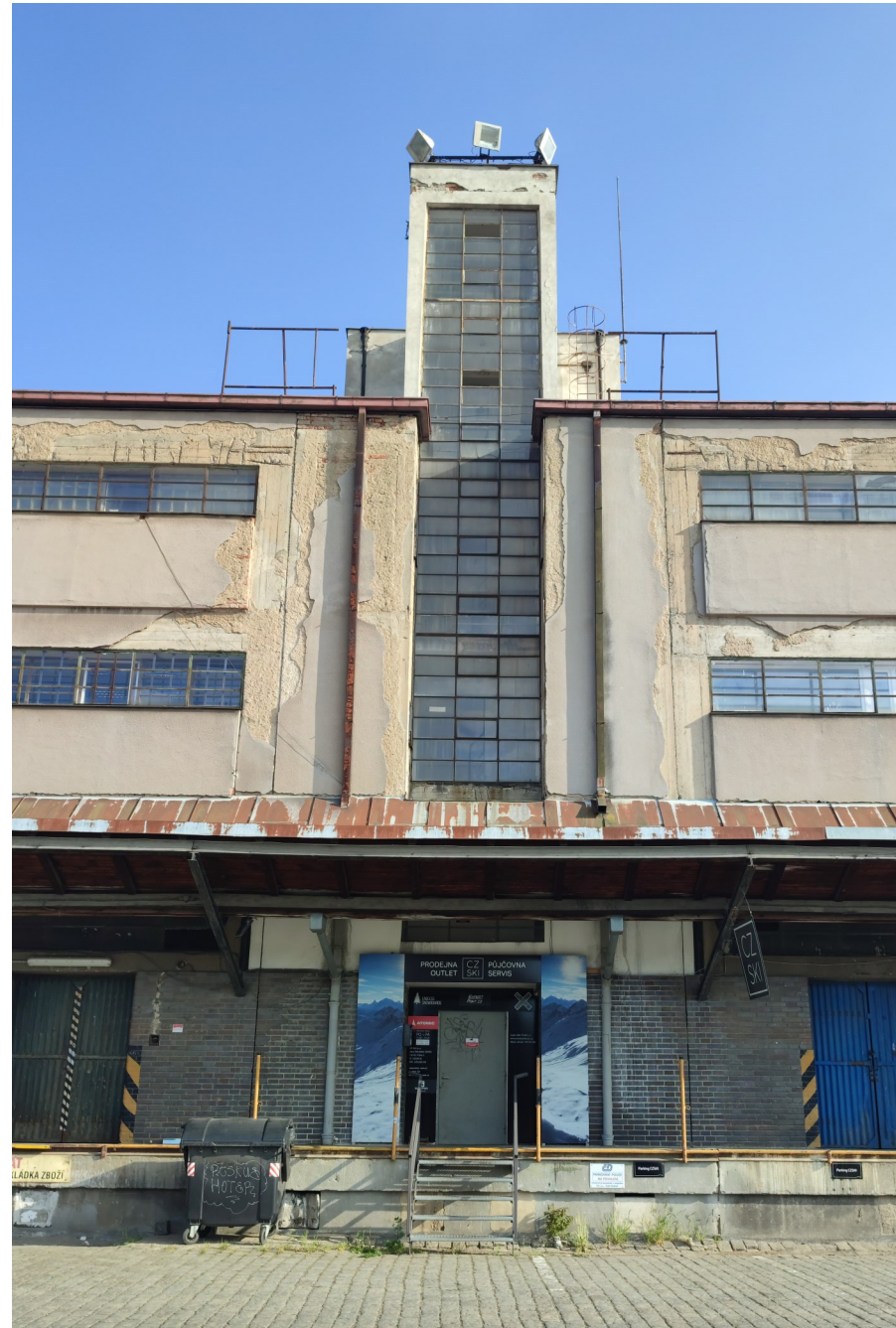
Image 18: North facade, staircase in the center.
