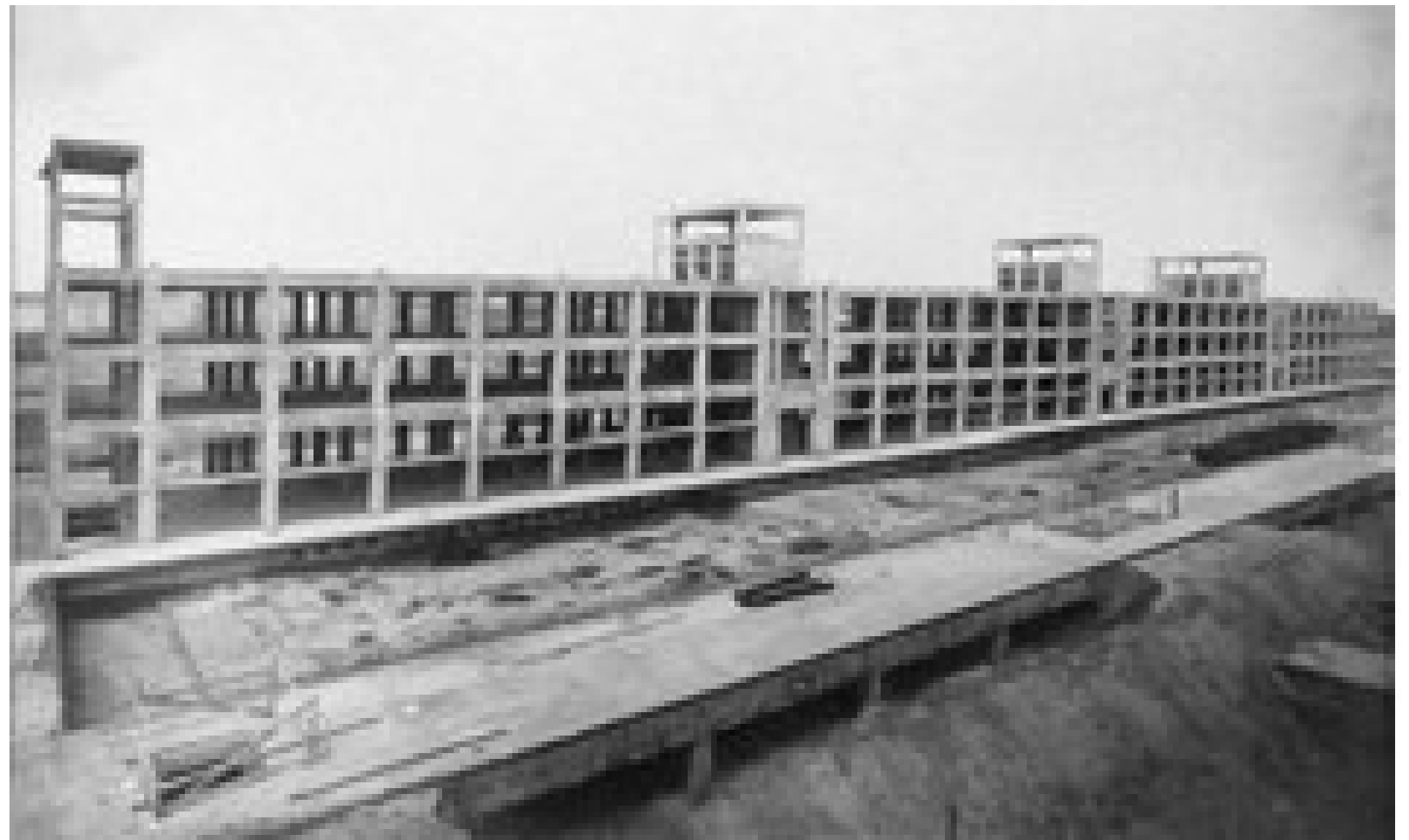
Image 8: Construction of the warehouse (north wing), 1933
