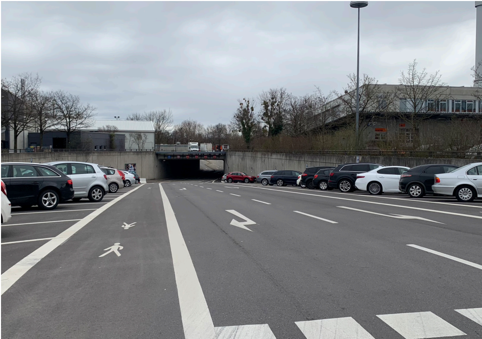
Figure 57: 5 Undersurpass in the area below the old railway line, west view
