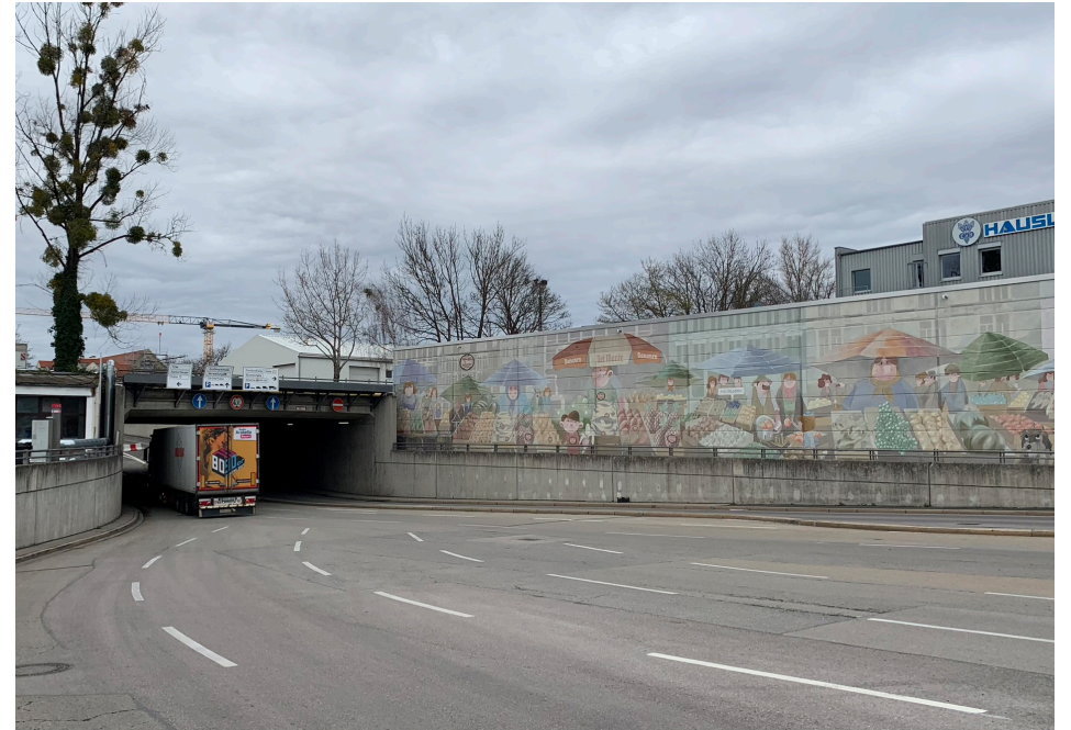
Figure 58: Undersurpass, east view
