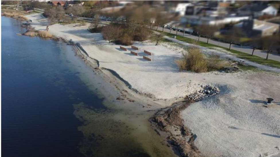
Figure 7. The results of the LIFE Coast Adapt project in 2021, showing with beach fences and beach nourishment on the BOJK beach (Lomma Kommun, 2023). Pictures used with consent.
