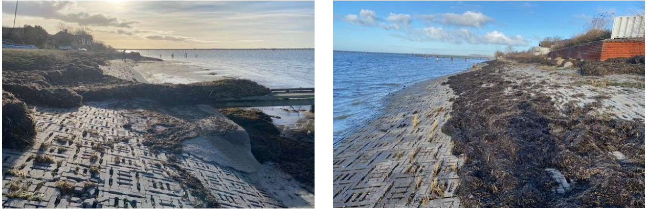
Figure 5. An example of the current grey coastal protection on two sites in Bjärred. Concrete tiles holding the shoreline intact. Pictures taken by the author. January, 2023.
