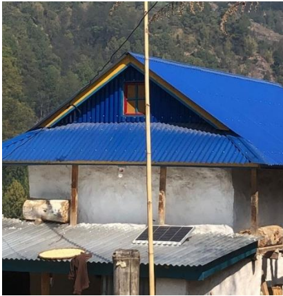
Figure 2 SHS on a roof. Photo taken by author.
