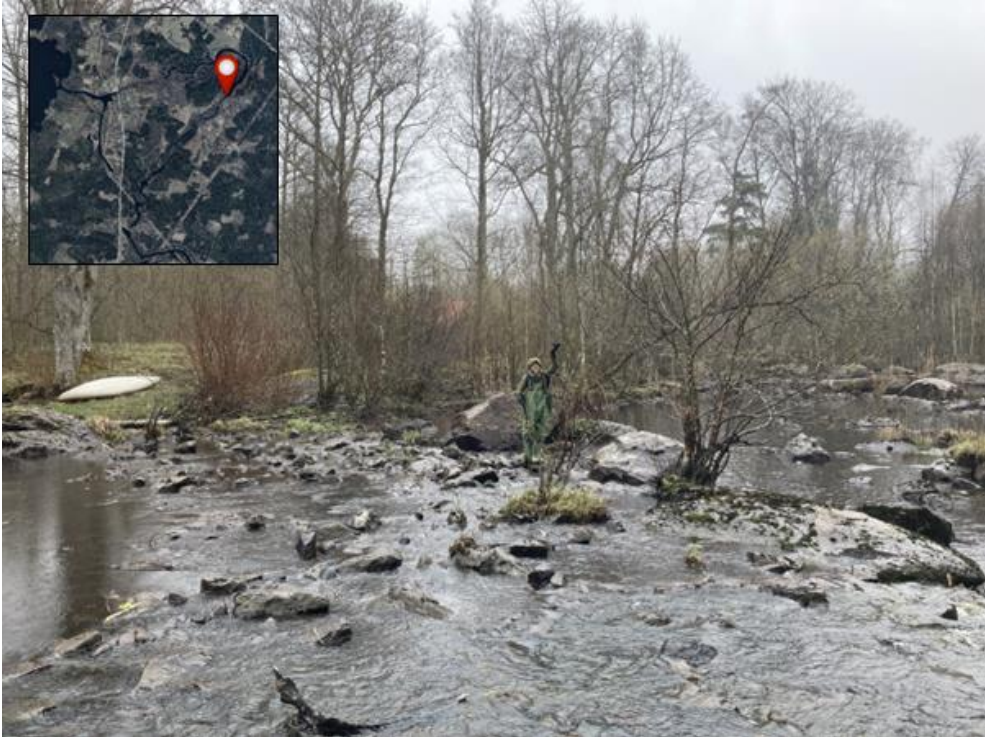
Figure 7. Göta dam, i.e., the rubble embankment dam upstream of Göta Bruk.
