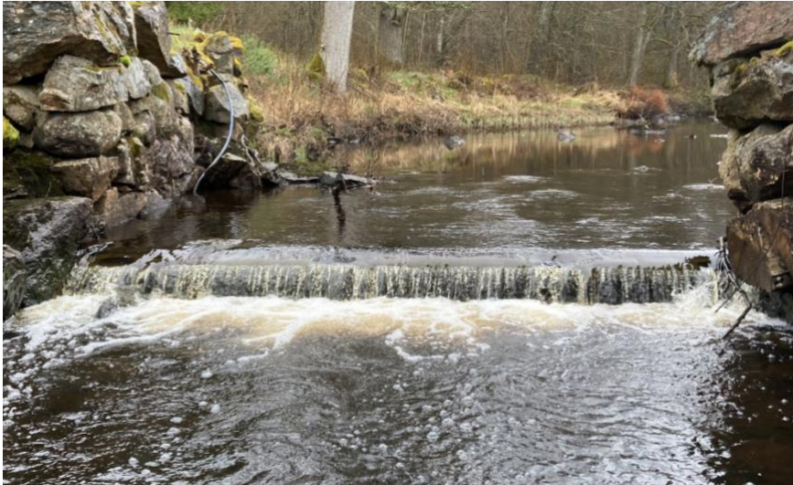
Figure 15. A small waterfall at the top of Göta bruk channel; potentially an obstacle for migratory fish.
