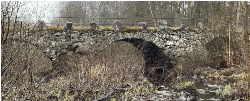
Figure 10. Photo of Knut's bridge, facing downstream. It has four arches, one outside the left side of the frame.
