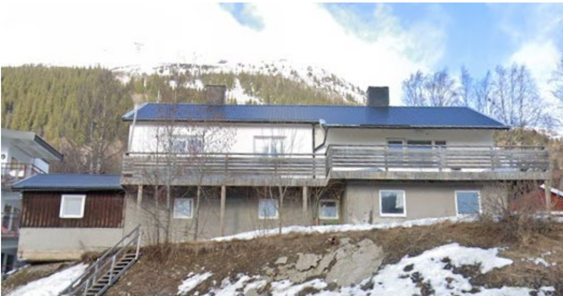
Figure 2 Picture of the south-facing facade of the case study building. Picture obtained from Google maps
