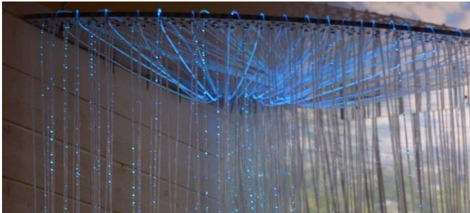
Figure 25 - Fibre optics pulled through a plexiglass plate to relieve stress (Komikapp, 2023)
