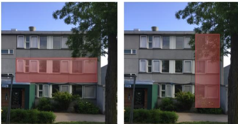
Figure 8. illustrate the attachment of the prefabricated facade onto the existing building facade and indicating a better illustration of how the windows need to be inserted in the prefabricated façade.
