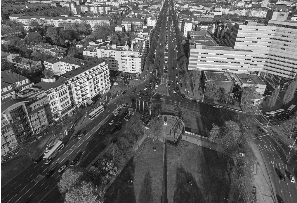
Figure 43: Teodor-Heuss Platz, aerial photo.
