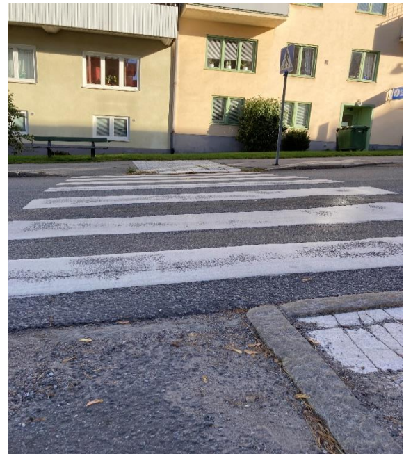
Figure 2.2. Crosswalk with curb cuts (Wigen, 2023).
