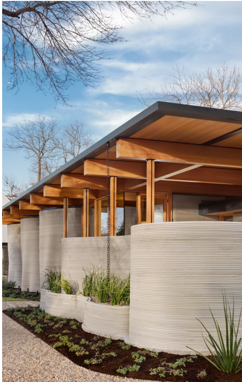
Fig 3.1 3D printed concrete House Zero by ICON. (House Zero 2022)
