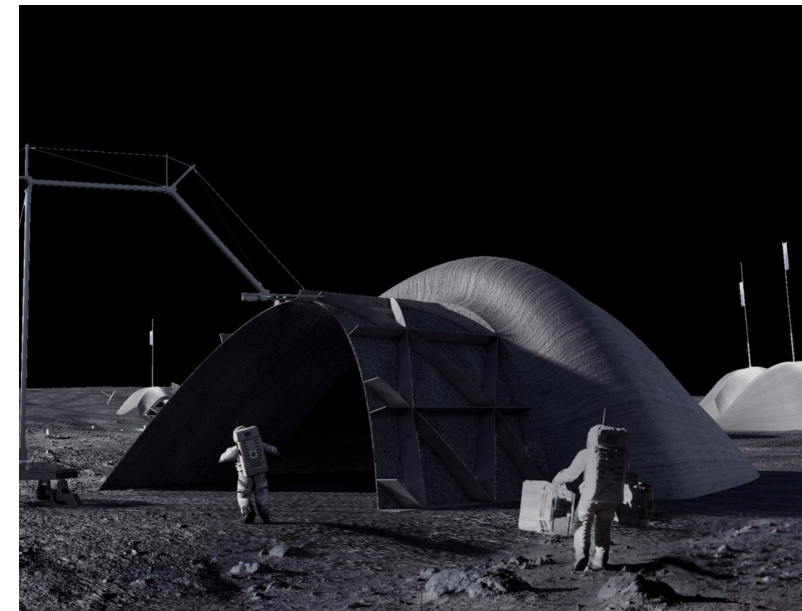
Fig. 3.2 Lina. 3D printed lunar structures by AI Spacefactory. (AI Spacefactory, Lina)
