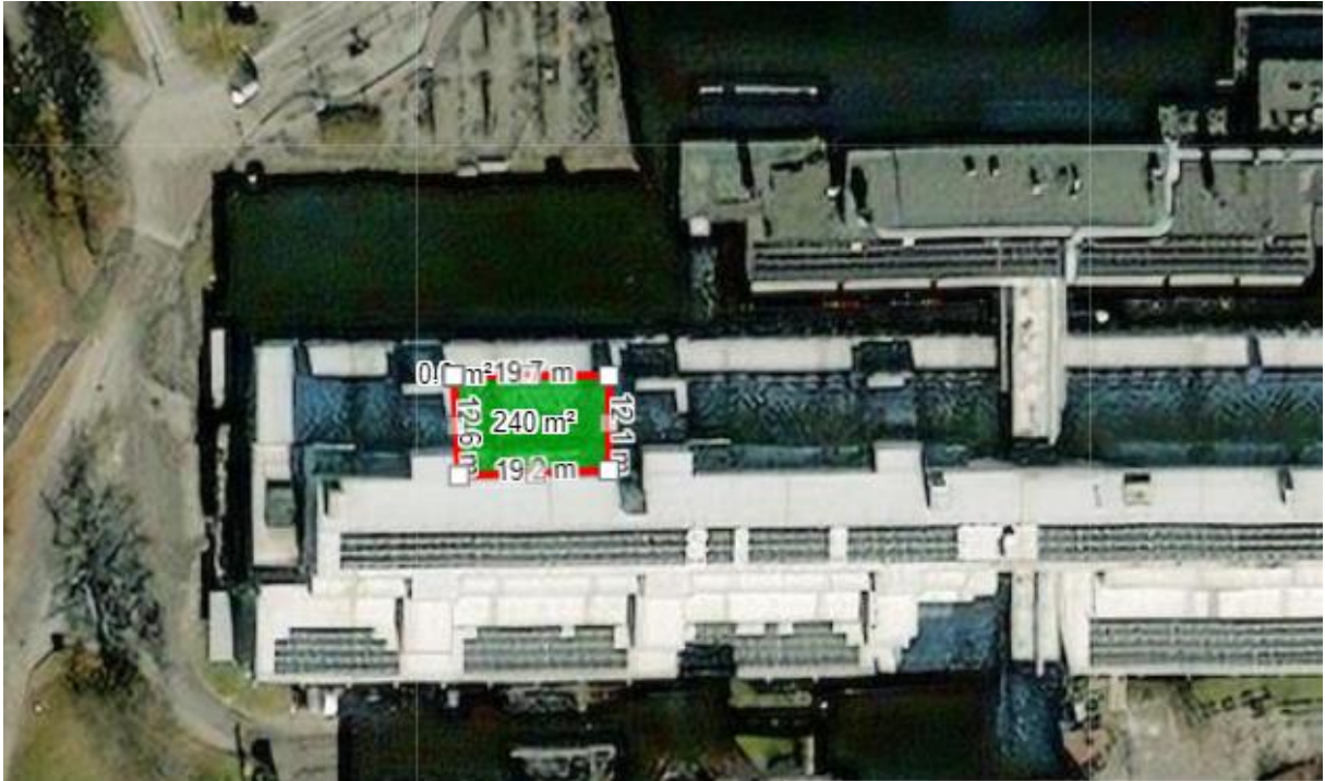
Figure 4.3. Rain collection area on the roof of Kemicentrum. Picture drawn in Daftlogic.com's Google Maps Area Calculator.
