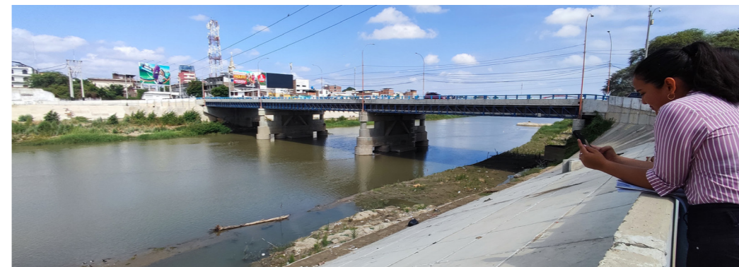
SANCHEZ CERRO BRIDGE Car priority
