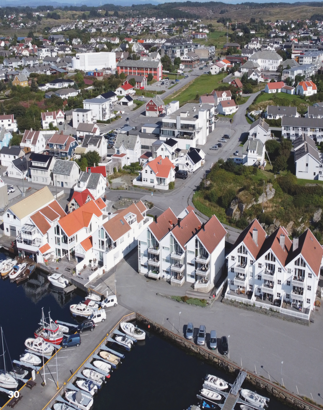
Figures. 13-17 Current images of Buildings and Conditions in Åkrehamn (Europan 17)
