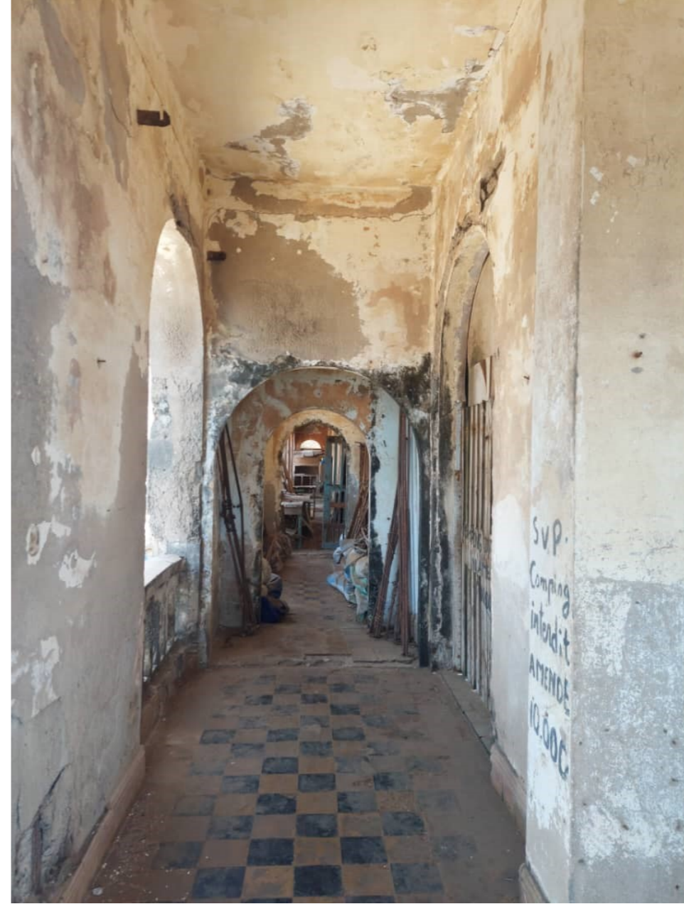
Left Upstairs gallery and room Roume Palace
