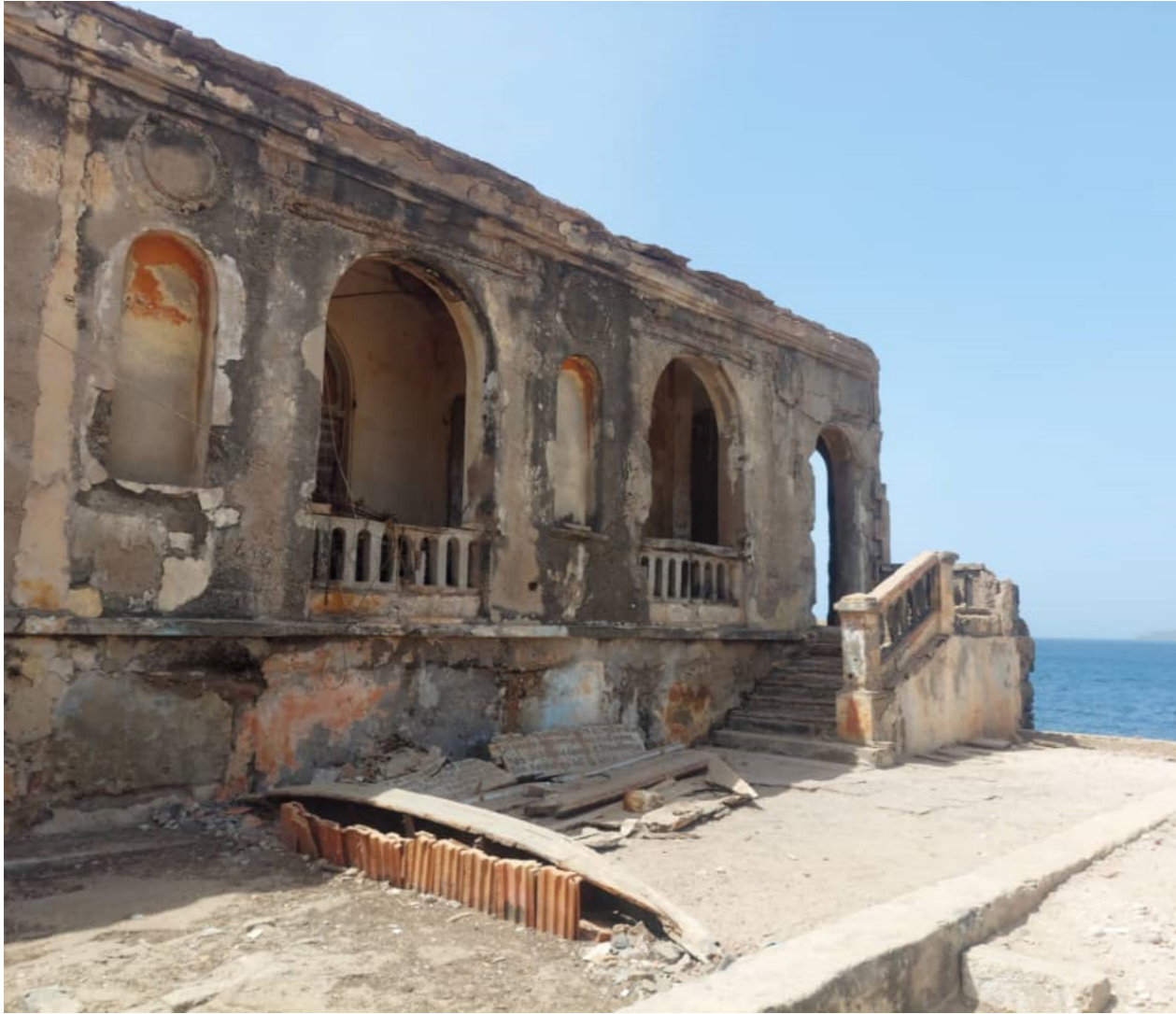
Annex building stairs to the terrace
