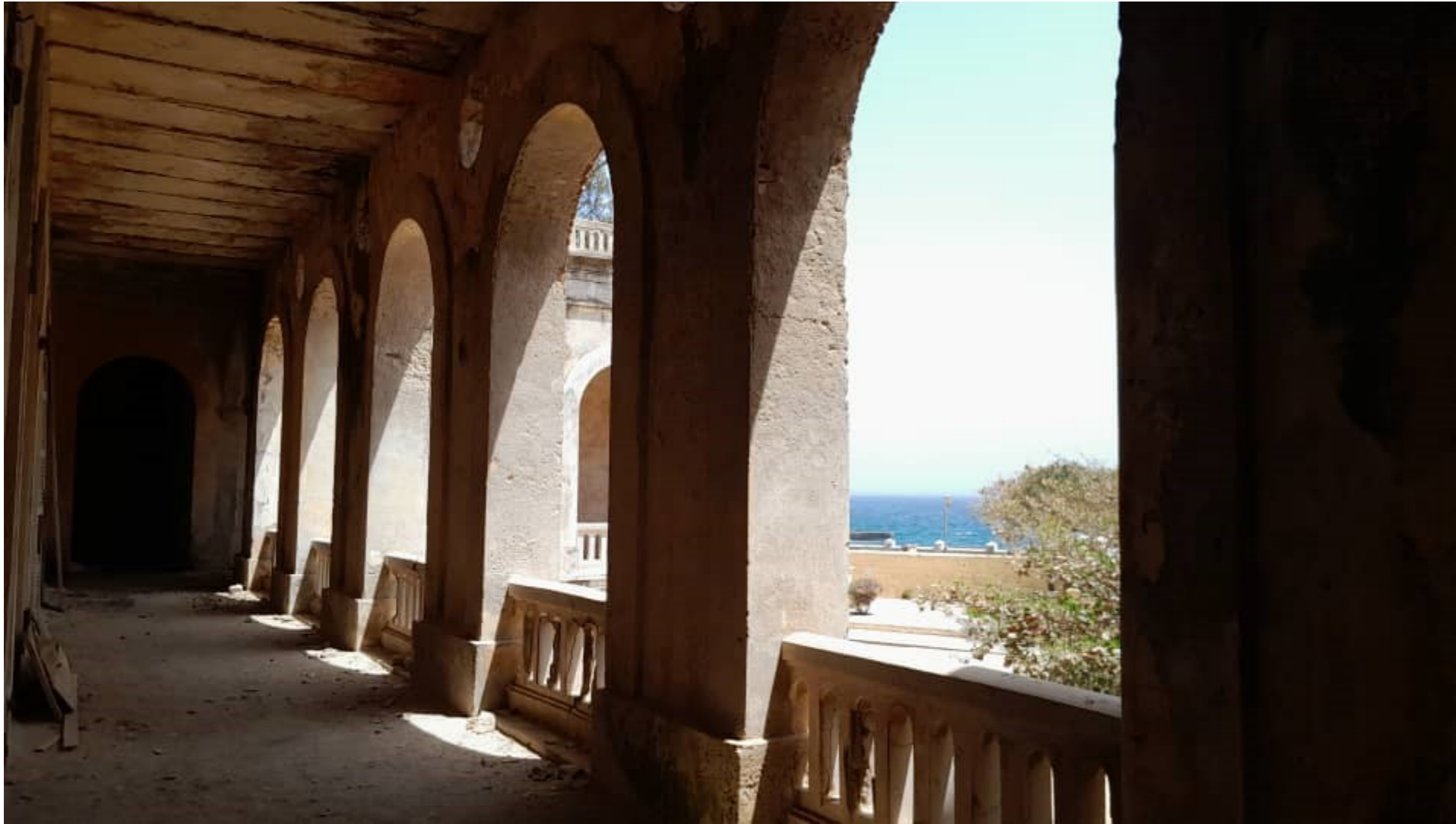
First floor arcade Roume Palace
