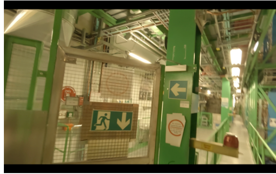
Figure 5.8: Emergency exit sign near visitor platform
