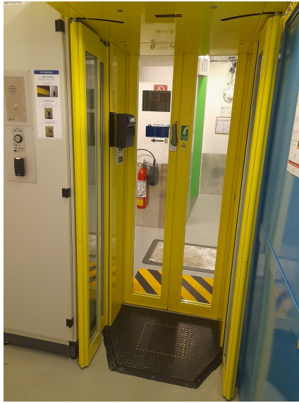
Figure 2.4: Personnel Access Device (PAD)
