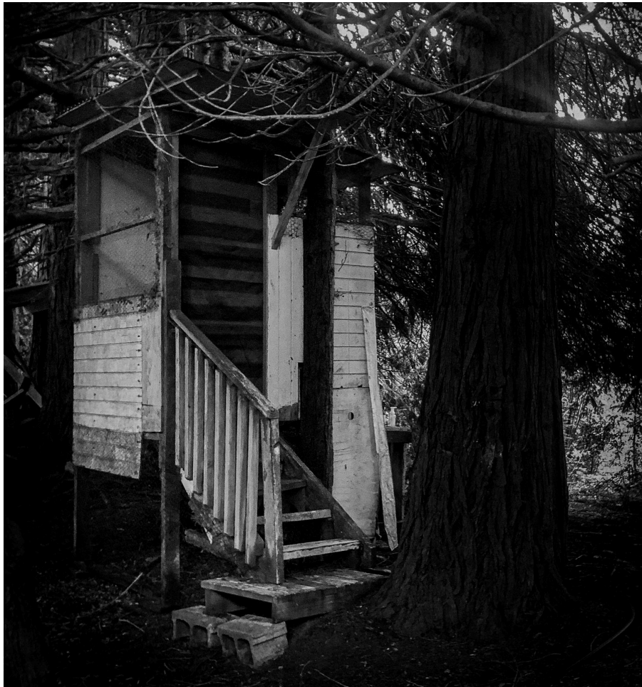
Figure 3. Composting Toilet - Exterior. Photo Sebastian Carlsson 2024.
