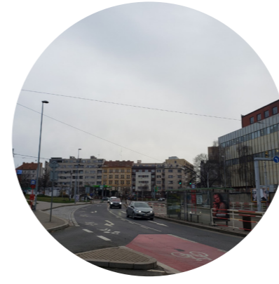
4. large, unsafe road
