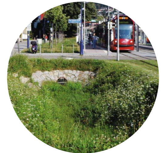
Central storm-water swale in Vauban. Photo: Thomas Schroepfer and Christian Werthmann, with Limin Hee
