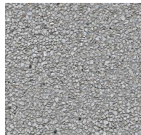
Exposed Concrete Walls
