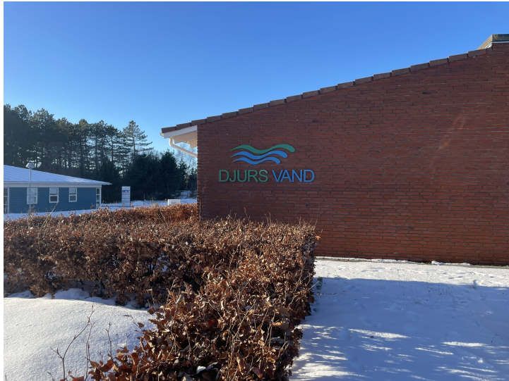
Figure 4.4. Djurs Vand office in Ebeltoft
