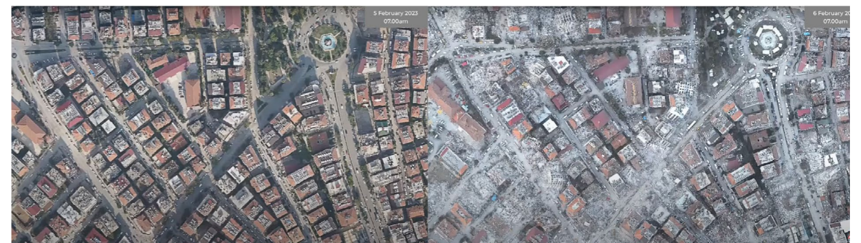
Fig4: Hatay, before and after the earthquake
