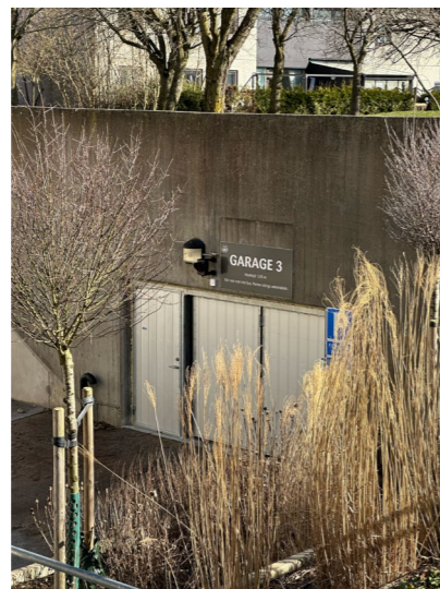
The entrance of underground car park
