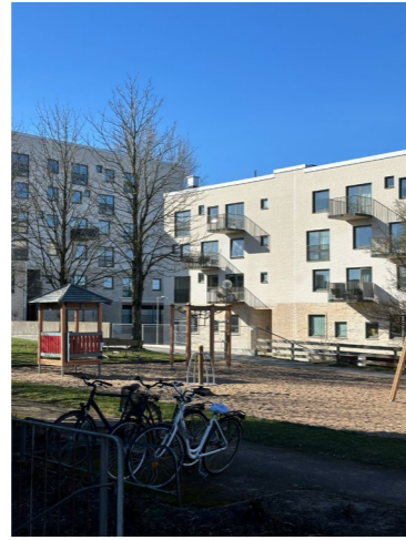
The playground & bicycle parking
