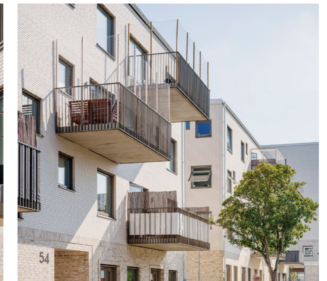
Fig.35 : A view from the facade
