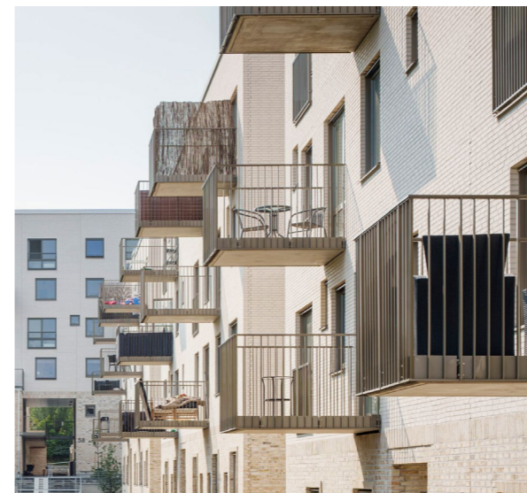
Fig.34 : A view from the facade
