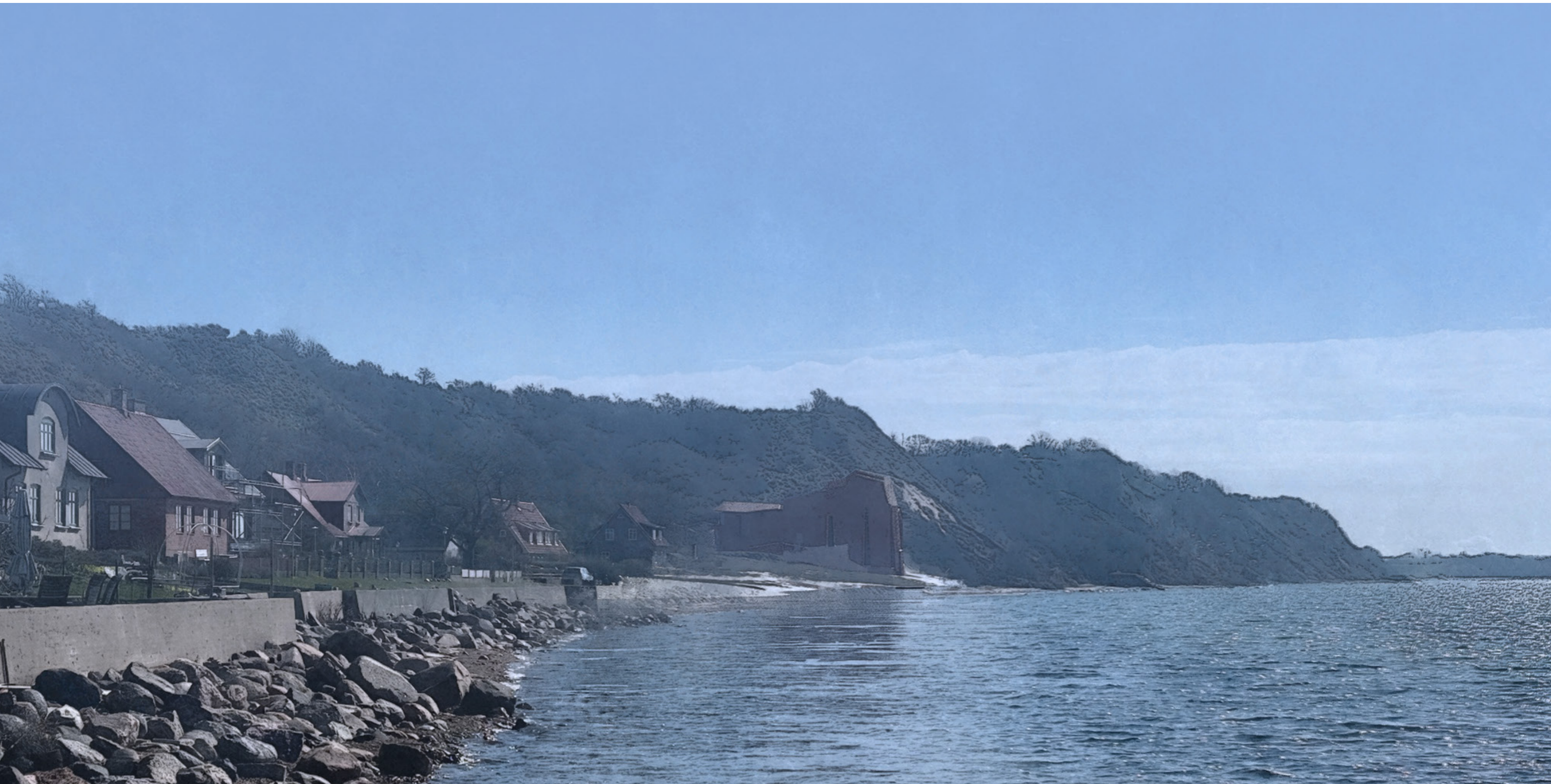
View from north
