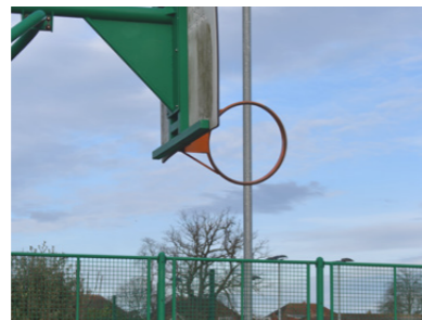
The cage has not been well maintained
