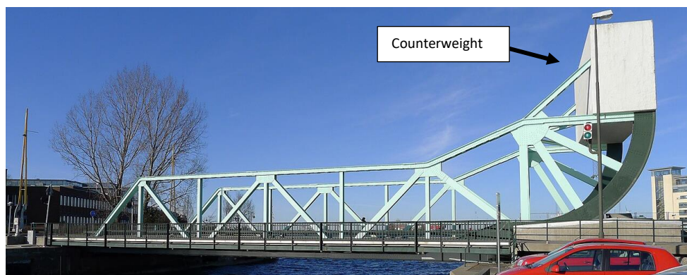
Figure 8.9 The bascule bridge in Malmö. (23)
