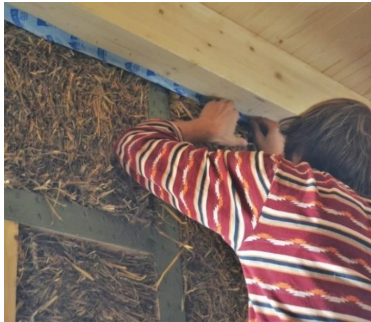
Figure 18: Application of building tape on the plaster - ceiling connection (ASBN, 2021)
