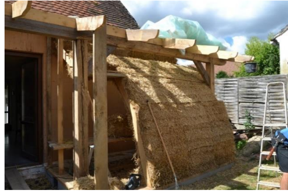
Figure 48: OrganiCUT Vault extension (Gruber, 2020a)
