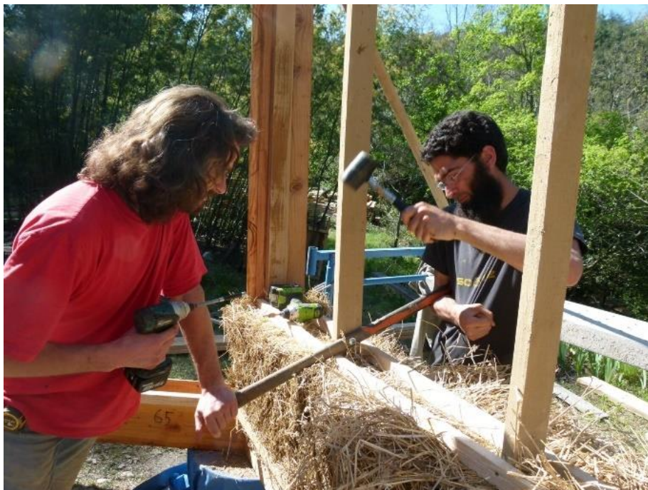
Figure 7: Compressing the bales in vertical direction with a lever machine commonly called “mammoth” (Rijven, 2024)
