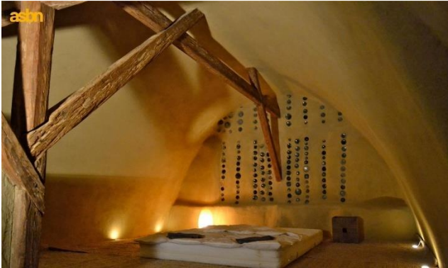
Figure 47: OrganiCUT in cold attic renovation (Gruber, 2020a)
