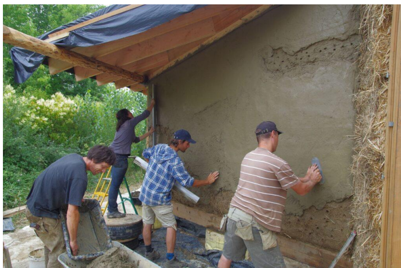
Figure 9: Smoothening the body coat with swimming pool trowel (Rijven, 2024)
