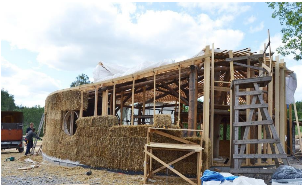
Figure 43: : OrganiCUT non-load-bearing CUT wall on the exterior side of the post and beam construction, Sweden (StrohNatur CZ, 2016)
