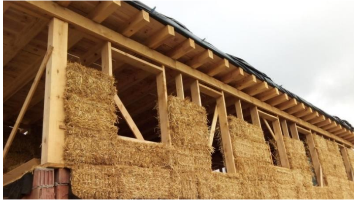
Figure 45: Load-bearing Post and Beam CUT (Toledo & Zecchetto, 2024)
