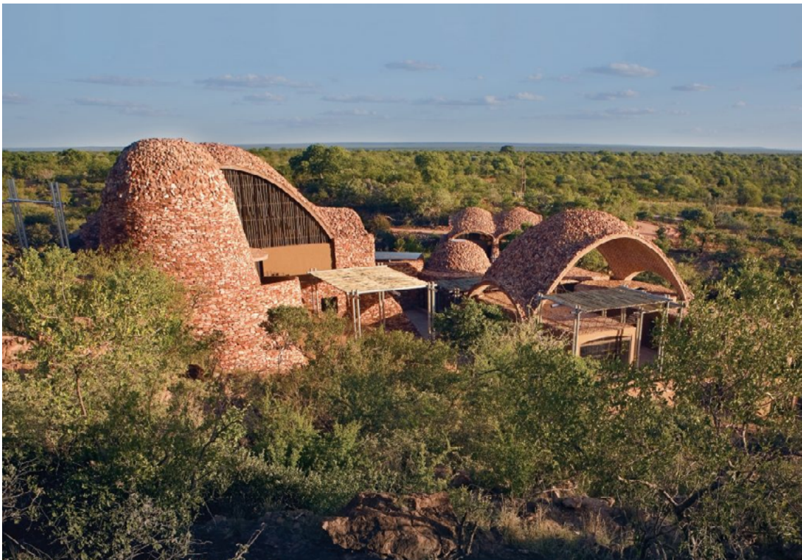
Figure 7 : Catalàn vaults in the Mapungubwe Interpretation Centre source: (Fagan, 2010)
