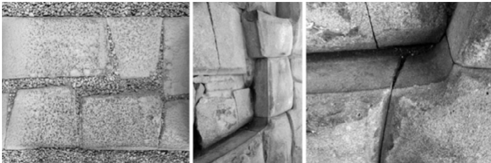
Figure 5: A series of Inca constructions that reveal the voided wedge between stones _ source: (Clifford et McGee, 2015)
