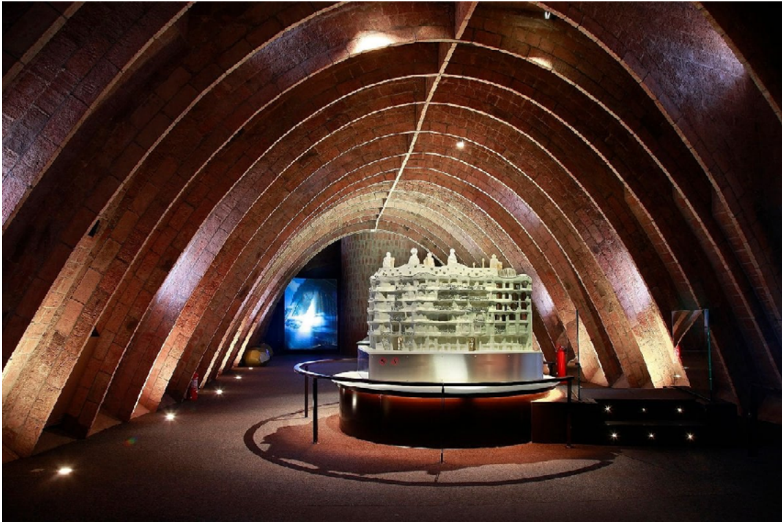
Figure 6: The attic from La Pedrera or Casa Milà by Gaudi, made of catalàn vaults source: (Jordi Play, s.d.)
