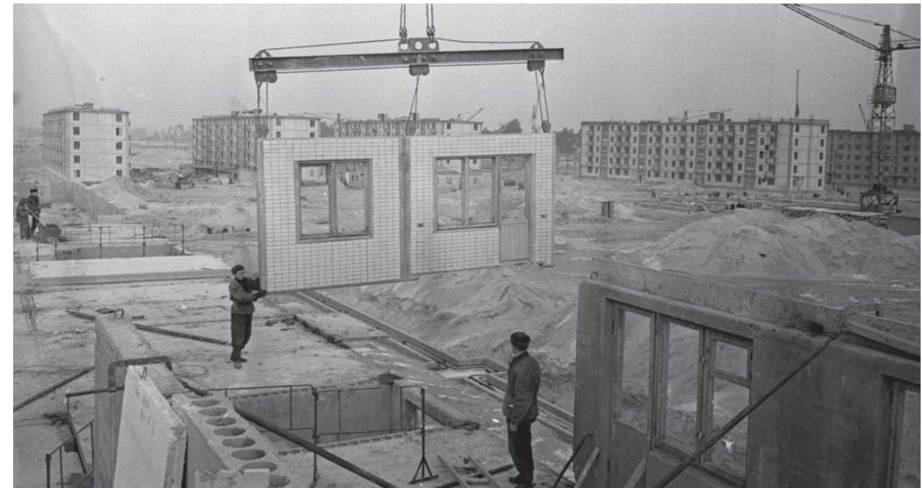
Fig. 4. Construction process of prefabricated buildings in the Soviet Union.
