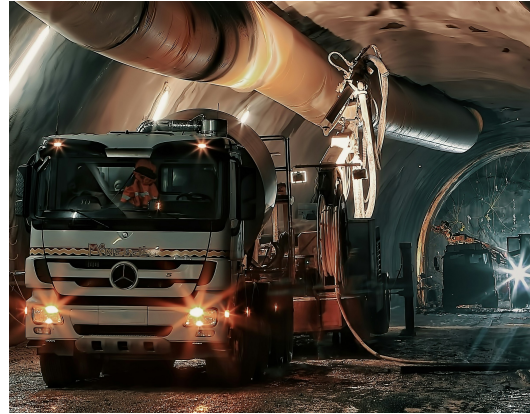
Figure 2.2: Example of an automated shotcrete robot, image by MTA Construction & Development Mega Projects [5].
