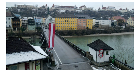
Figure 27: Bridge towards Burghausen
