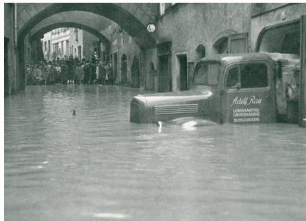
Figure 23: Flooding of an Street in the old town
