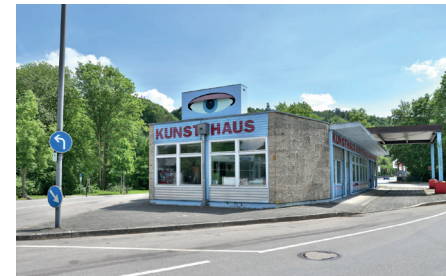
Figure 26: Border controllhouse on one of the bridges
