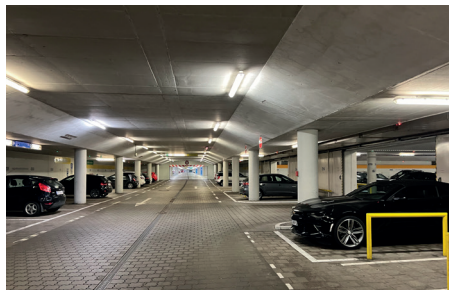
Figure 105: Picture of the underground parking
