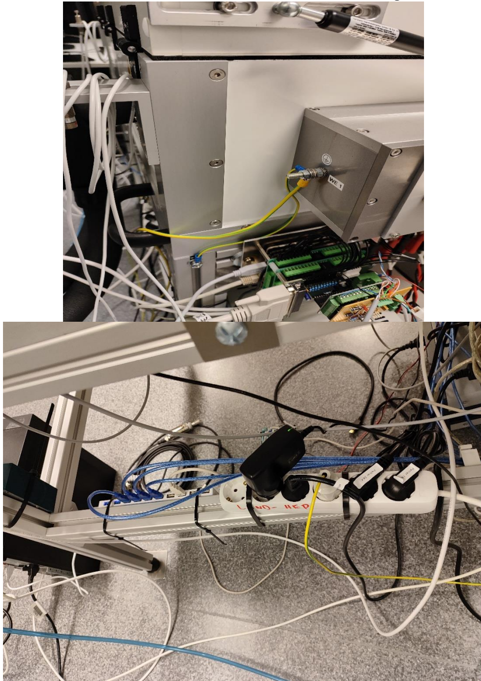
Figure 18: Grounding of the box.
