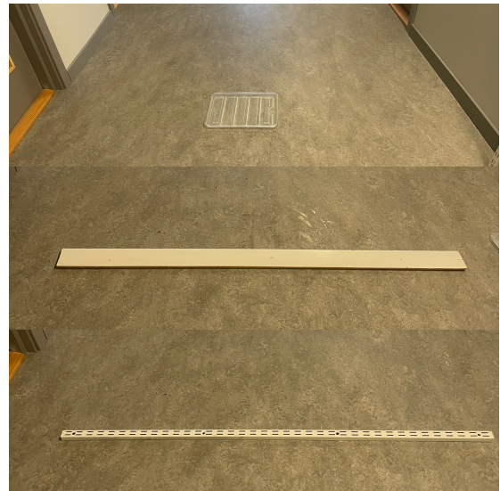
Figure 9. Water pit, wood threshold, metal threshold
