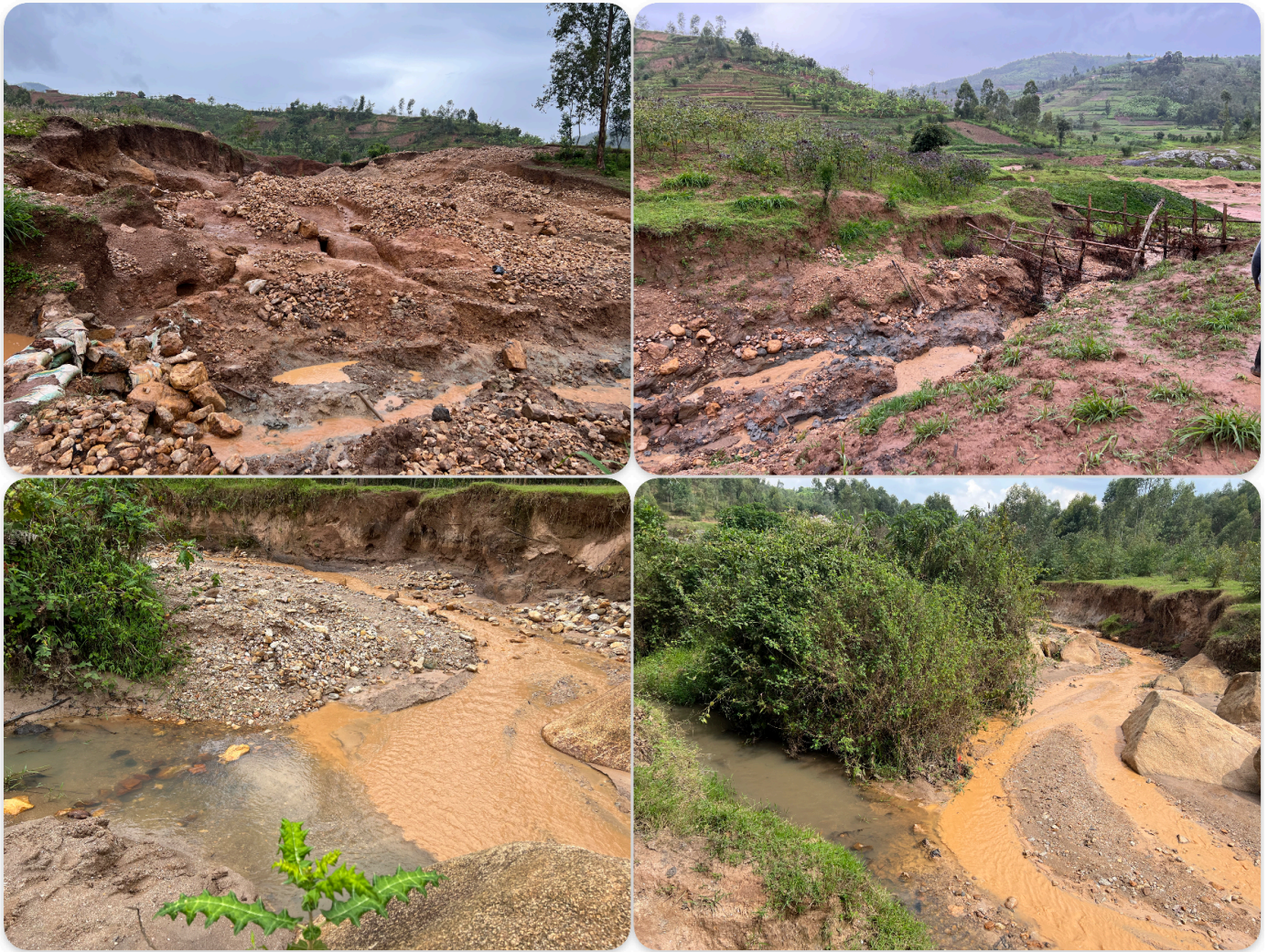
Figure 4.13 Impact from mining activity in Nyagako catchment. Top pictures: Mining site in Zone C. Bottom left: Junction between outlet from A1 and A2 in Zone A. Bottom right: Junction between A3 and upstream mix of A1 and A2 in Zone A.
