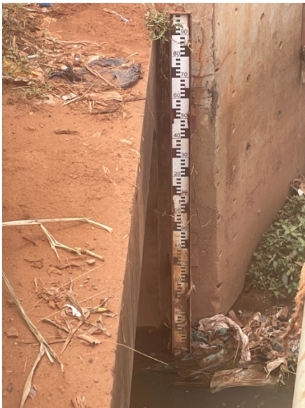
Figure 9 Water level meter located on a box culvert along Hoima Road.
