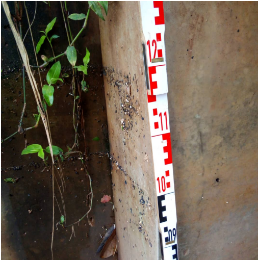
Figure 10 Peak indicator of water level on culvert.
