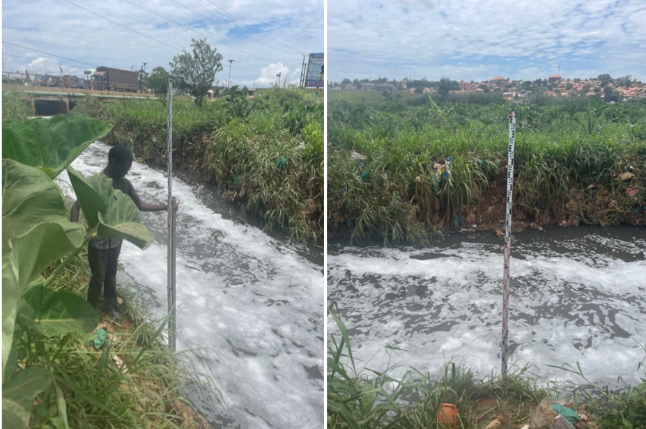
Figure 8 Water level meter located in the Lubigi main channel.
