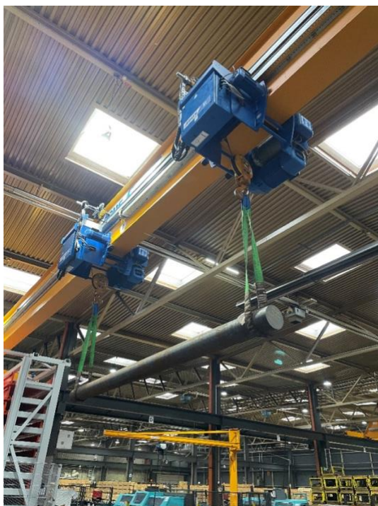
Figure 43: Overhead crane transportation
