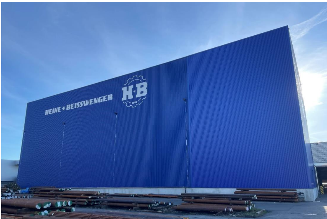
Figure 38: High rack warehouse of Heine + Beisswenger.
