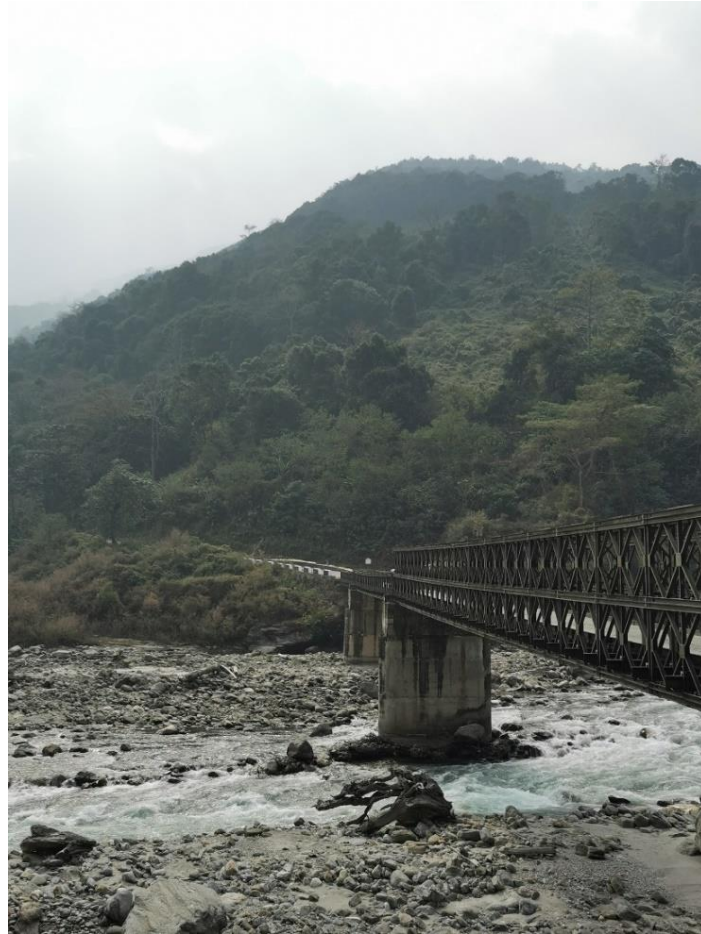
Figure 8: Road Bridge Crossing Amo Chu River (personal photo)
