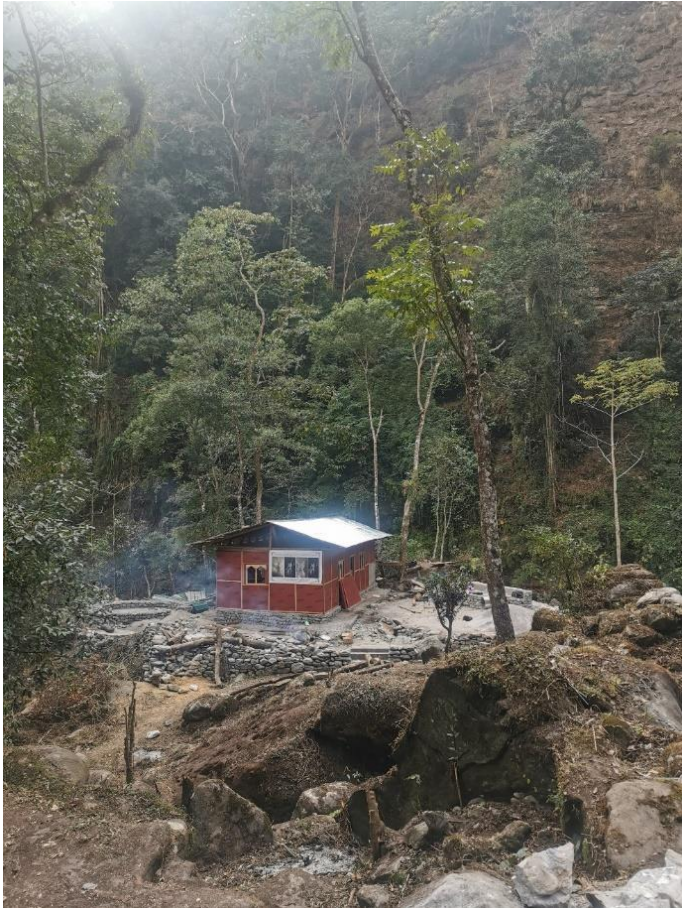
Figure 13: Sales Counter and Hot Stone Bath under Construction at Rangtse Nye (personal photo)
