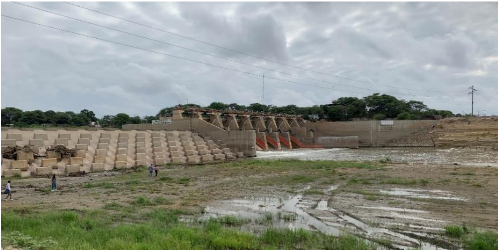
Figure 24- Los Ejidos dam spillway
