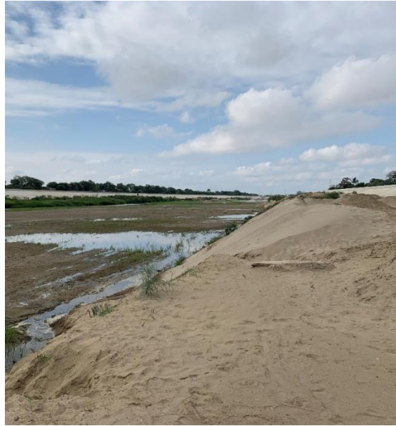
Figure 6- Sediment build up at Los Ejidos view from top
