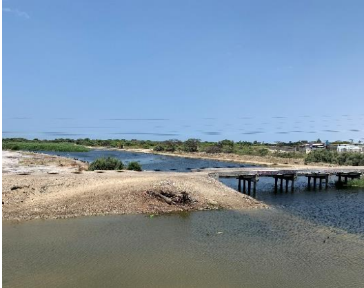
Figure 49- Downstream view at Sechura Bridge
