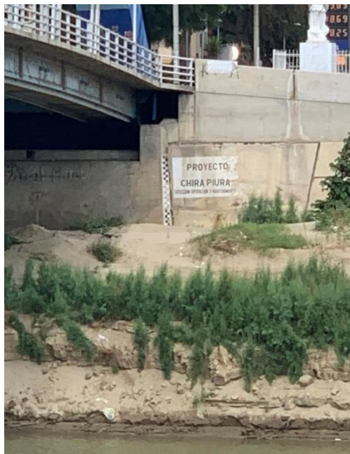
Figure 19- Gauge at Bolognesi Bridge
