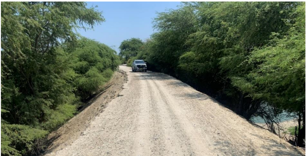
Figure 42- Dike bordering Lagoon
