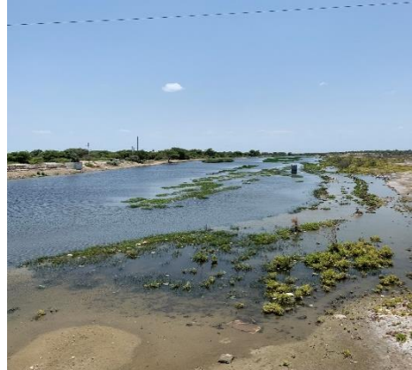
Figure 50- Upstream view at Sechura Bridge
