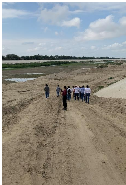
Figure 4- Ramp into the floodplain at Los Ejidos
