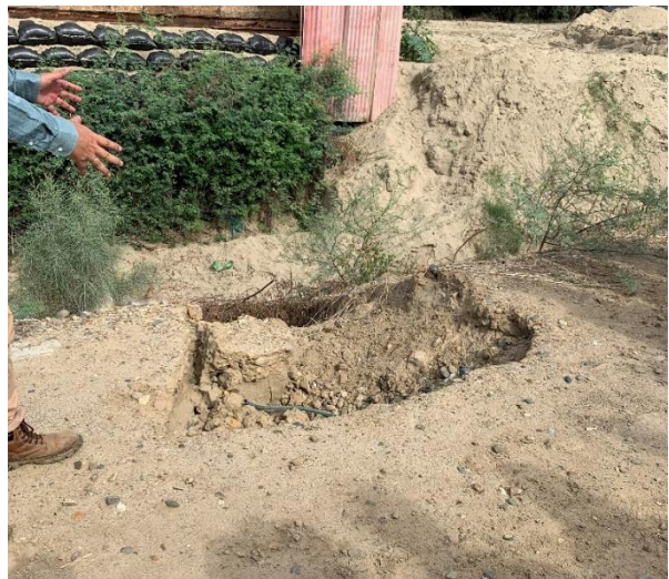
Figure 11- Hole on 'dry side' of riverbank
