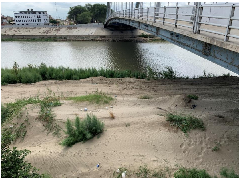
Figure 20- Below Bolognesi Bridge
