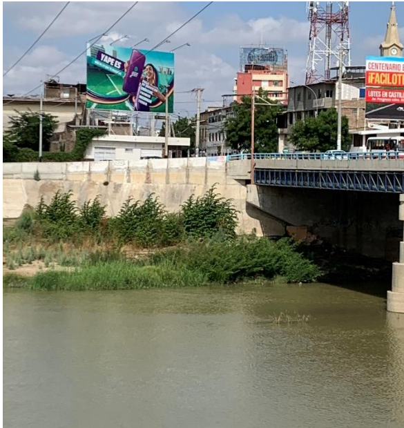
Figure 15- Below Sánchez Cerro Bridge
