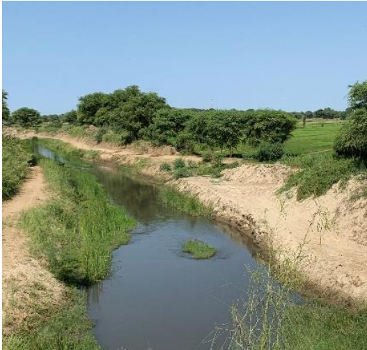
Figure 31- Drain 13.08 on right side of river
