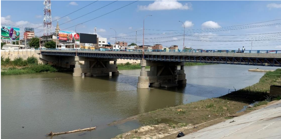
Figure 14- Sánchez Cerro Bridge
