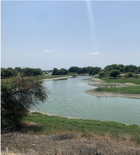
Figure 40- Upstream of dike, in Lagoon
