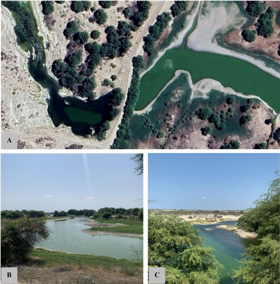
Figure 31a- Ñapique Lagoon dike (Google Earth, 2024). 31b- Upstream of dike. 31c- Downstream of dike
