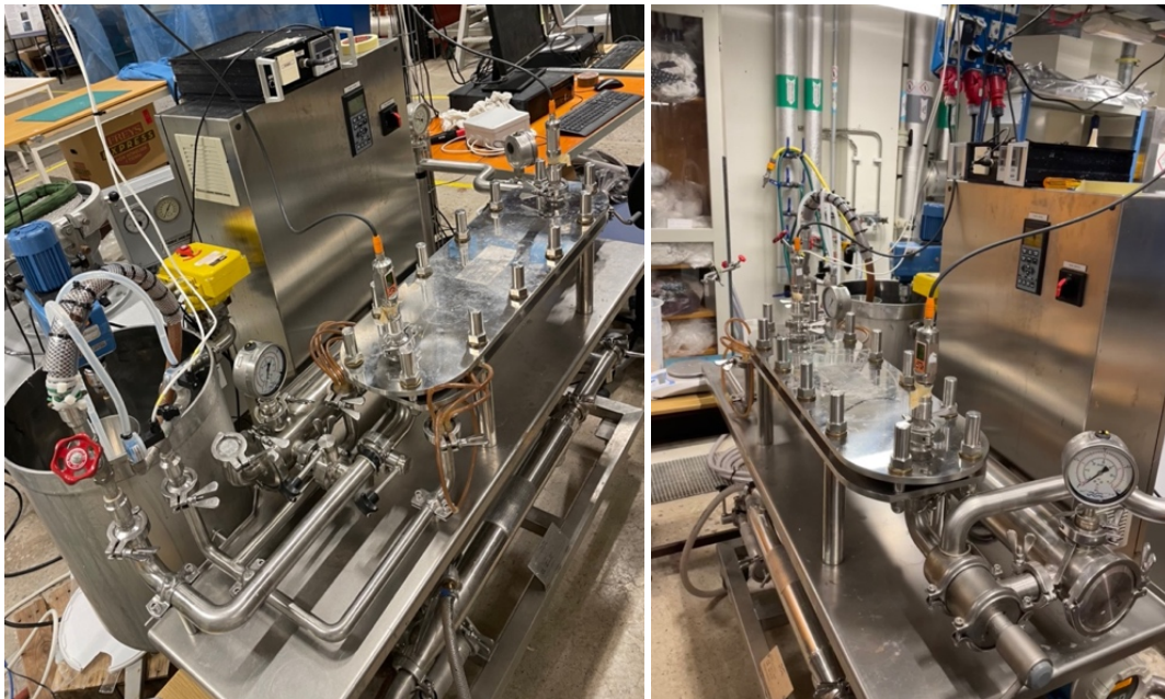
Figure 3. Membrane filtration system from Alfa Laval.
