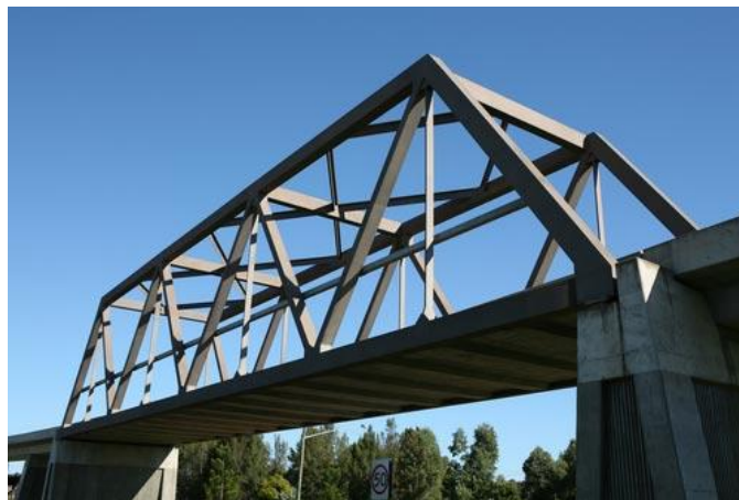
Figure D.10 Truss bridge (Bridge Masters, 2017).
