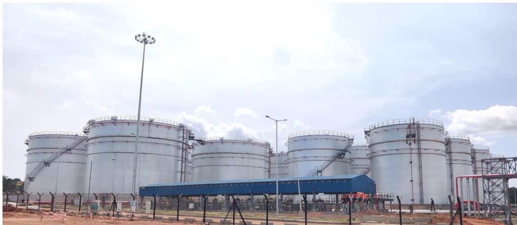
Fig 10: Fuel storage tanks at Mahathi Infra
