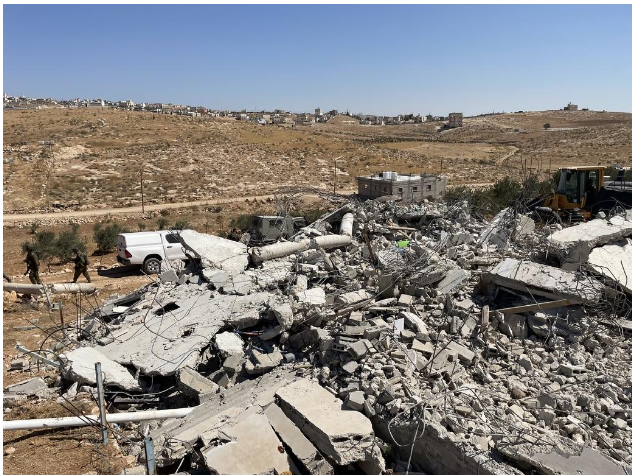
Figure 9: Demolished house in Jawaya by author
