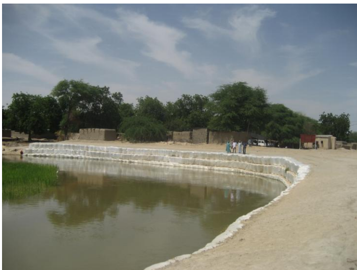
Figure 3.10. Reinforcement of the banks of the meander, by the local organization PADL, at Bosso.
