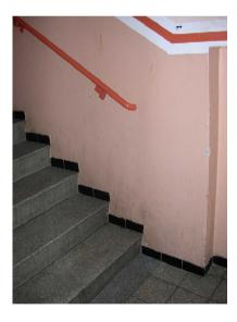
Figure 6. Two of the core environmental barriers identified. Letterboxes can only be reached via differences in level (left), and handrails are too short (right).
