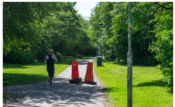
Image 19 - A warning of a cracked surface
