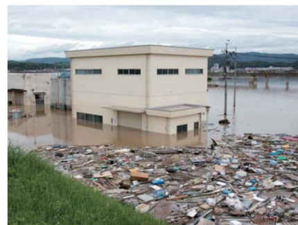
Household items washed away by muddy waters In the case of flood damage, not only household items but also earth, sand and sludge are washed along with the muddy flow and can become the cause of stench.
